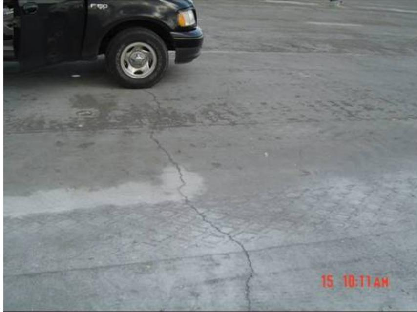
Figure 2-3. Shrinkage cracking in CTB.
