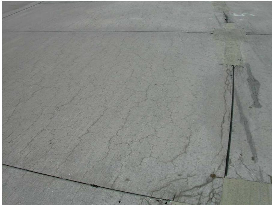
FIGURE 2. ASR DISTRESS IN CONCRETE PAVEMENT AT COLORADO SPRINGS AIRPORT
