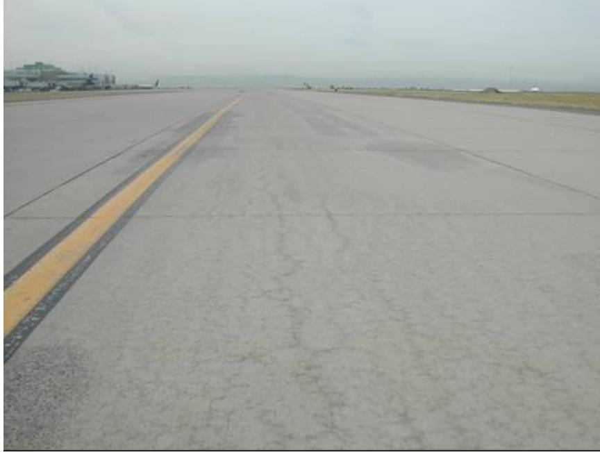
FIGURE 1. ASR DISTRESS IN CONCRETE PAVEMENT AT DENVER INTERNATIONAL AIRPORT
