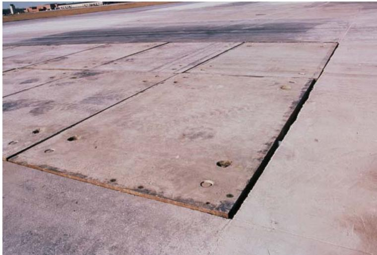
Figure 3-2. Temporary pre-cast panels at Savannah.
