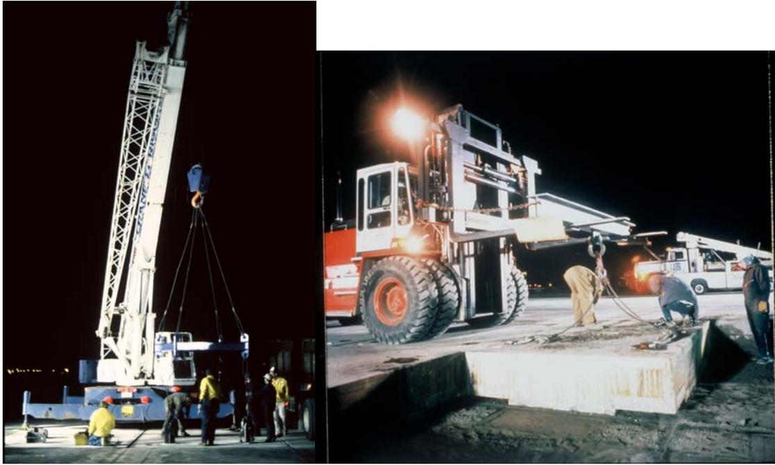
Figure 3-3. Larger crane used in Charleston (left) and smaller equipment used in Savannah (right) to place temporary pre-cast panels.
