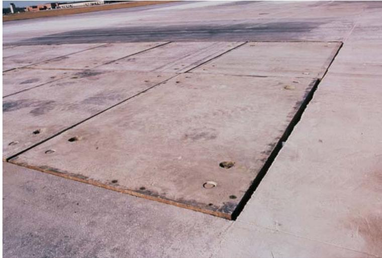
Figure 3-2. Temporary pre-cast panels at Savannah.
