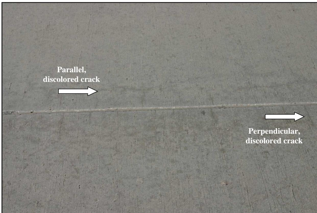
Figure 17. Example 3: tightly closed cracking along joint.
