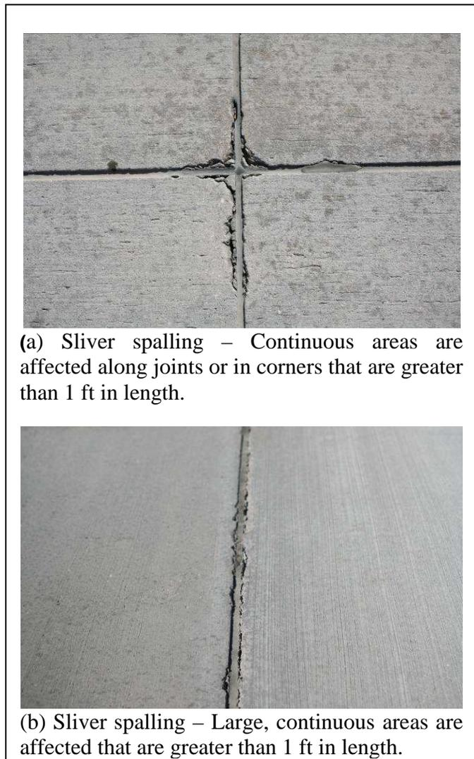
Figure 8. Sliver spalling.
