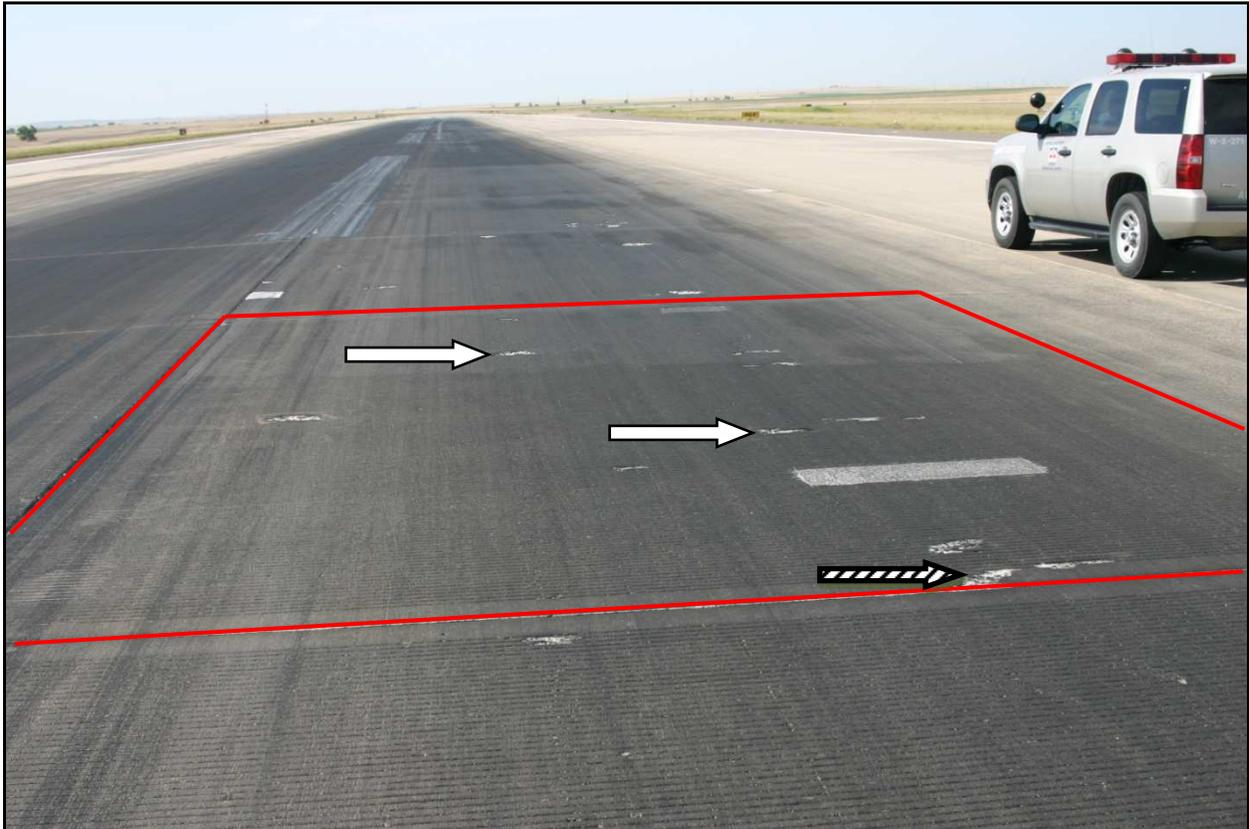
Figure 16. Example 2: interior of slab on runway touchdown zone blackened with tire rubber.
