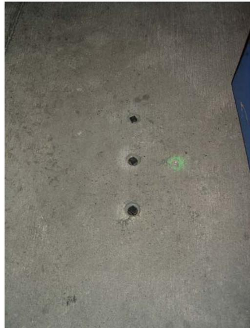
**Figure 9: Humidity Wells Installed (12" Top, 6" Center, 2" Bottom) at Phoenix Sky Harbor International Airport**
