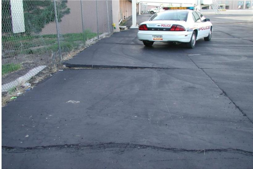
Figure 2-4 Heaving in an airfield pavement (Sarkar, Zollinger, and Mukhopadhyay, 2004).
