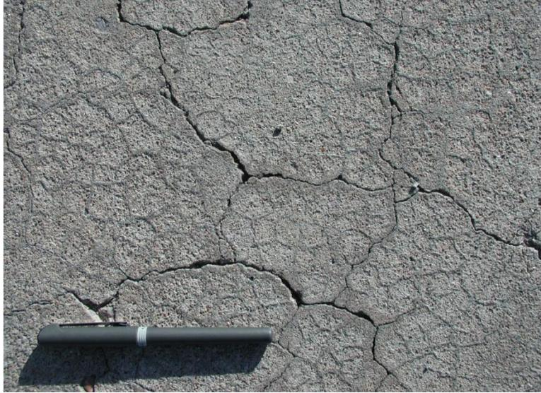
Figure 2-2 Map cracking, portion of an airfield concrete pavement (Sarkar, Zollinger, and Mukhopadhyay, 2004).
