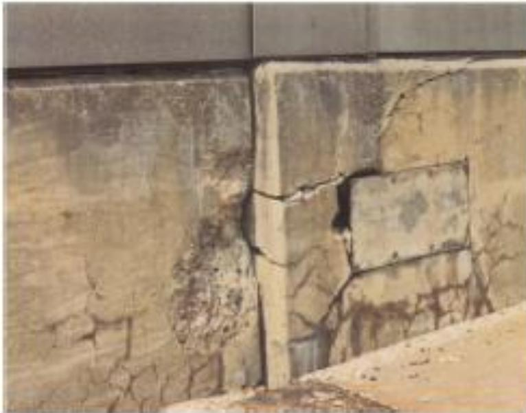
Figure 2-3 Misalignment of adjacent sections of a parapet wall on a highway bridge due to ASR (Strategic Highway Research Program (SHRP)-315, 1991).
