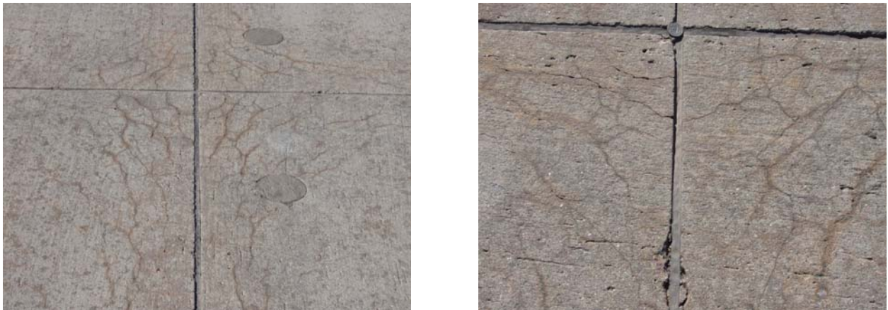
Figure 14. Surface condition of pavement in airport B
