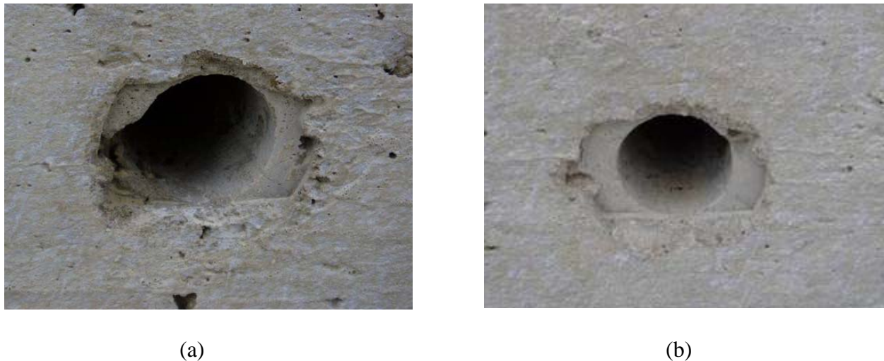
Figure 9. Dowel holes created using plastic sleeves: (a) result where the horizontal hydraulic jack snagged; (b) result where the equipment functioned properly.
